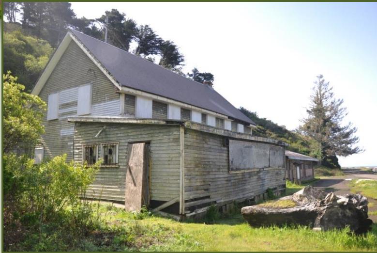
1948 bar addition beginning to collapse in 2010
