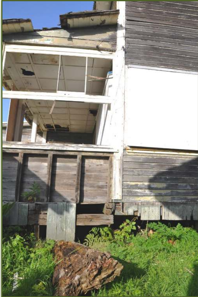
Foundation structure completely rotted away
