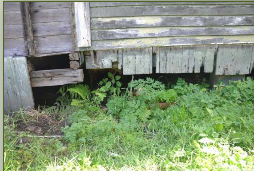
Foundation structure completely rotted away
